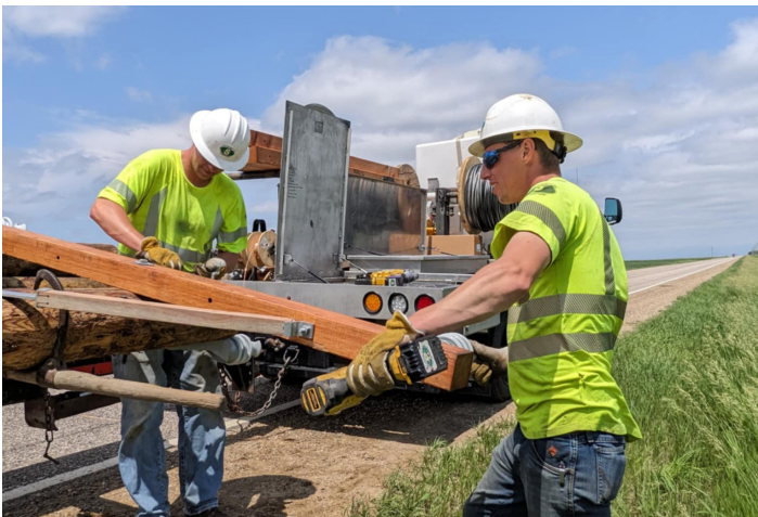
Line crews work to replace a power pole following a 2025 storm.
