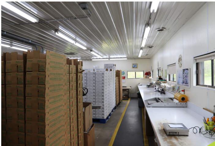
Lights in the packaging area were retrofitted to LEDs.
