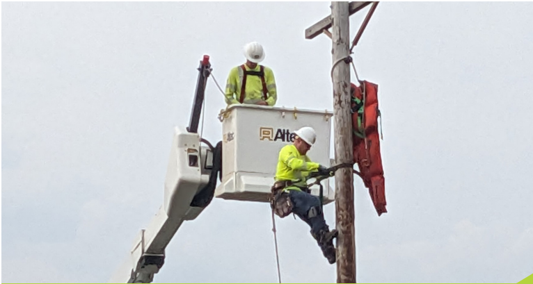
Lineworkers complete pole top and bucket rescue training annually.
